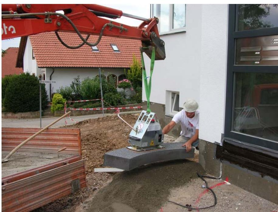
Universal, battery driven Vacuum Laying device to install non porous concrete or natural stone elements up to a max. of 400 kg. Here installing rounded step elements, weight each about 200 kg.
